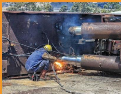
Roof support section being dismantled
