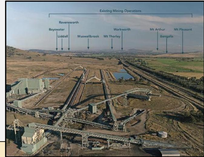
Substantial infrastructure in place including CHPP, rail loop, conveyors and wash plant. Operations to be day shift only to minimise community disturbance.
