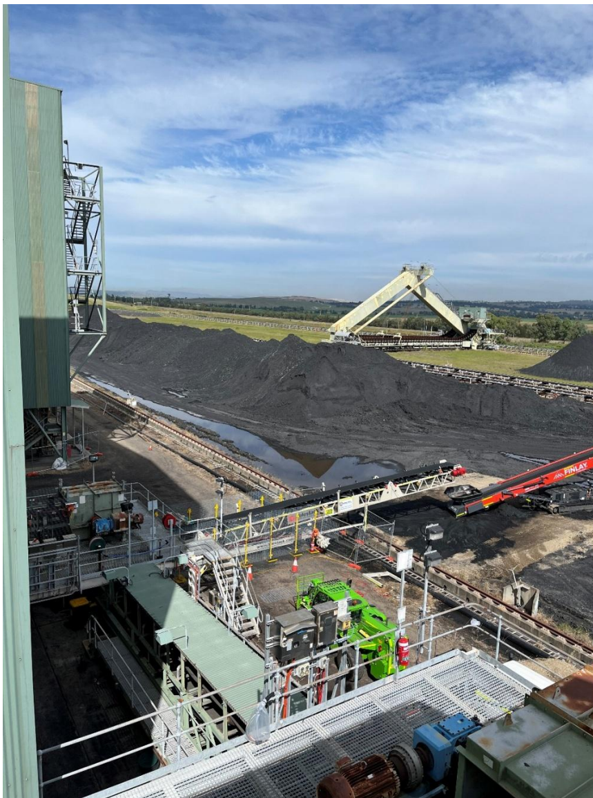
Dartbrook Coal Handling Preparation Plant (CHPP)
